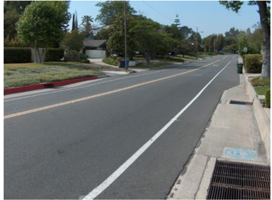
Installation of Class III Bikeway signing.
