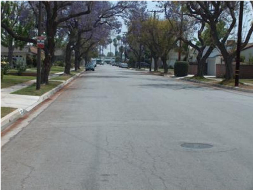
Installation of Class III Bikeway signing, “Share the Road” signs and Sharrow pavement legends.
