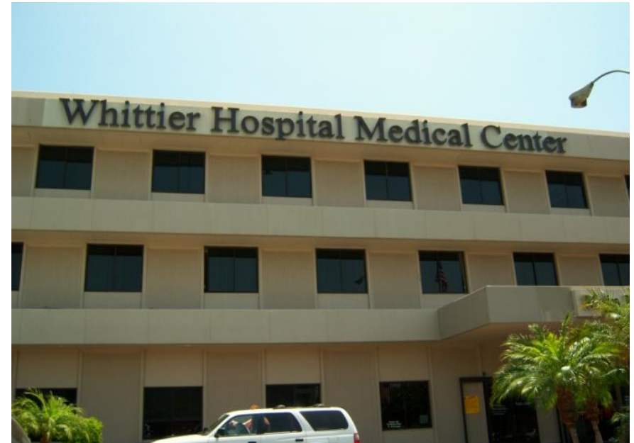
Whittier Hospital Medical Center, directly accessible from Colima Road (Class II) and future Class III on Janine Drive.
