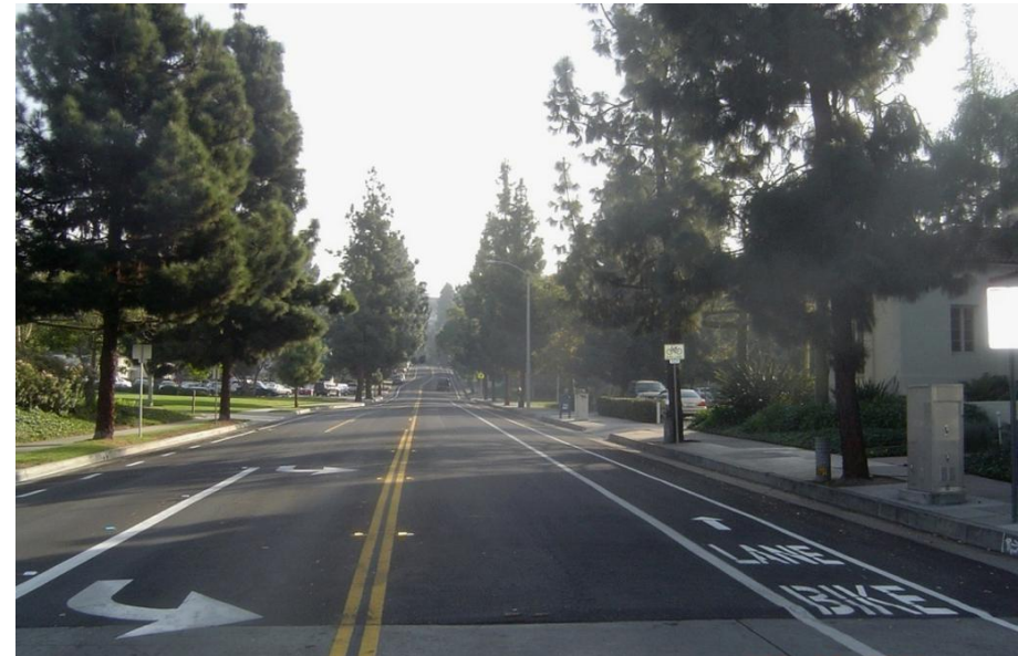
Upgraded Class III Bike Route with striping of Class II Bike Lanes adjacent to the campus of Whittier College.
