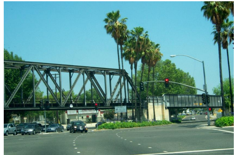
Whittier Greenway Trail continues on bridge deck over Whittier Boulevard at Five Points
