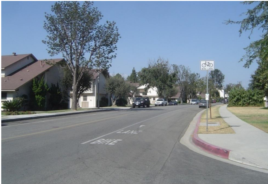
Striping of northbound Class II Bike Lane and installation of “Share the Road” Signs with “Sharrow” pavement markings for the southbound Class III Bikeway.
