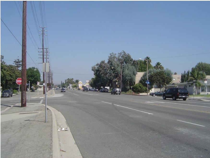
Upgrade of Class III Bike Route with the installation of Class II Bike Lanes.
